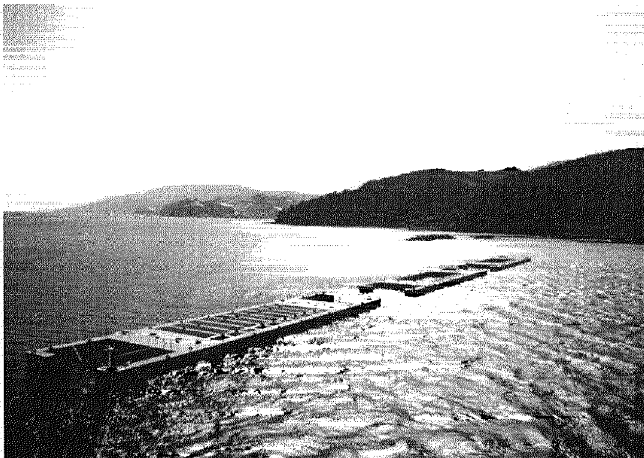
Figure 6. The floating breakwater
