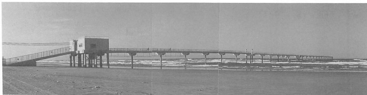
Figure 2. Photograph of the Hasaki Oceanographical Research Facility. The beach slope is flat, and the width of the surf zone is more than 200 m. This is the typical dissipative sandy beach.
